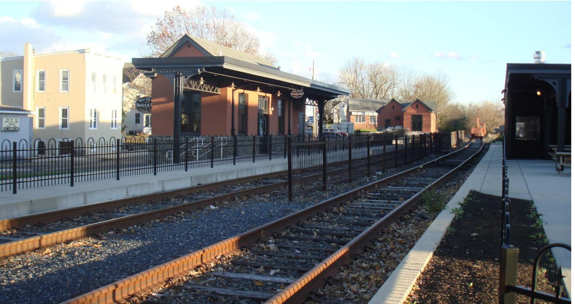
Historic Buildings at the Souderton Train Station, refurbished for reuse by local businesses.
