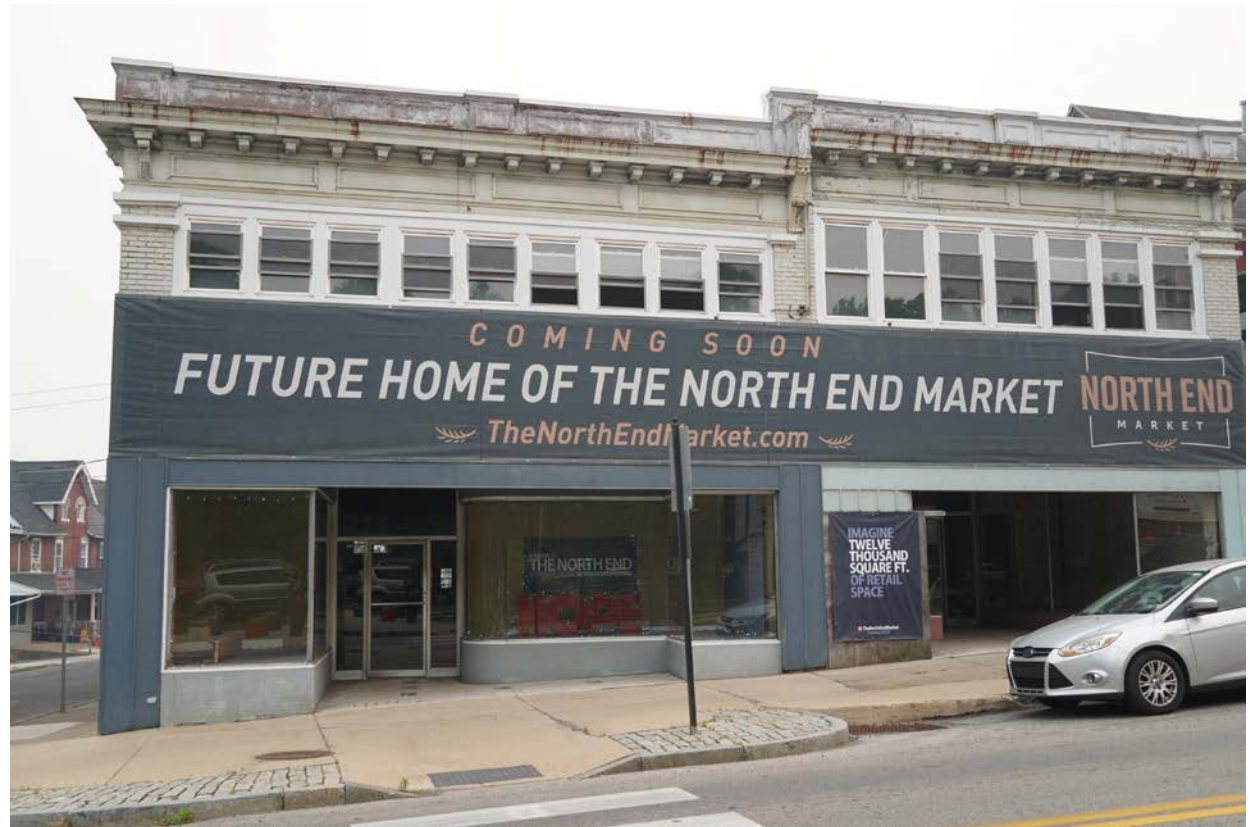
The historic R. E. Hope clothing factory and store is slated to become North End Market.
