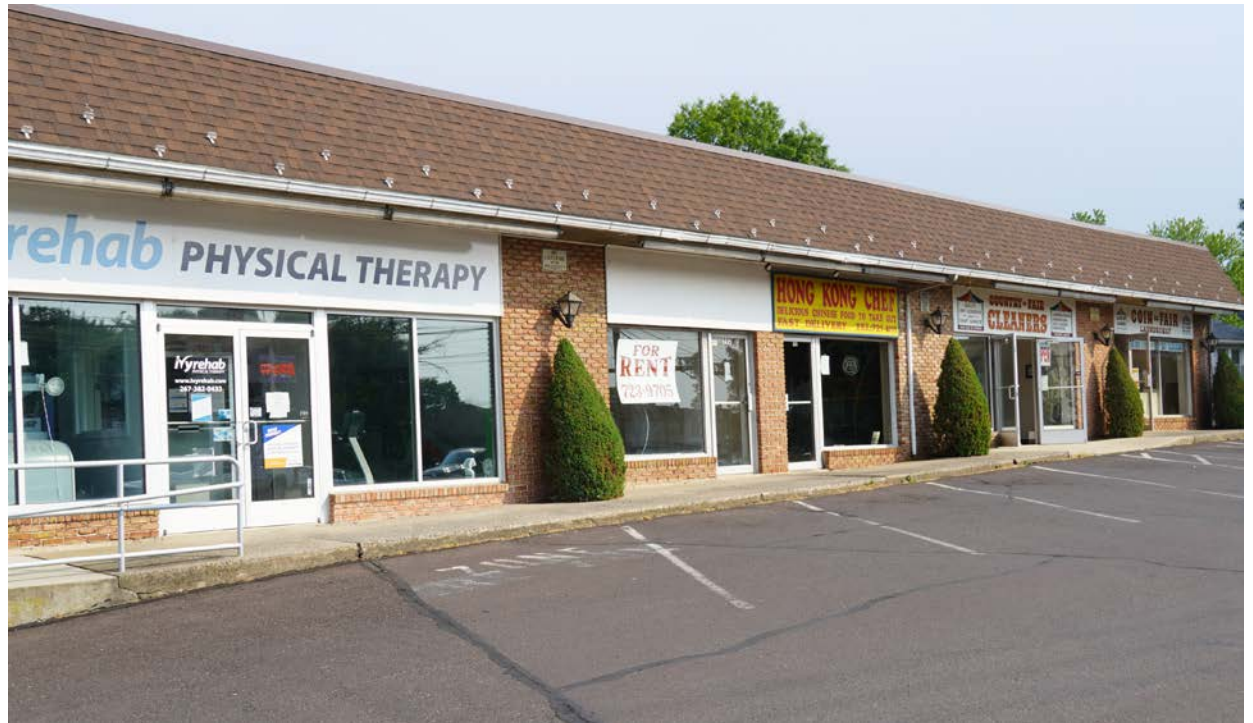
A vacancy in the shopping center on Broad Street at School Lane.
