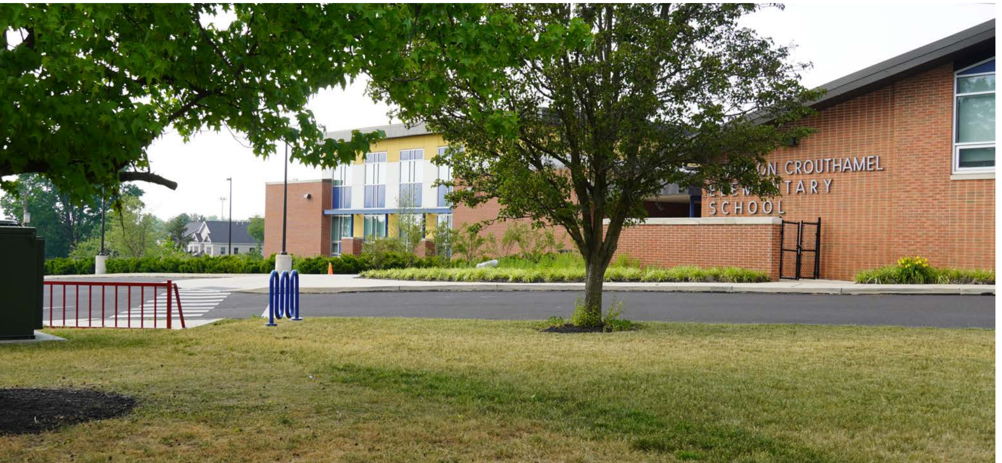
E. M. Crouthamel Elementary school in 2023; the new portion of the building is on the left.
