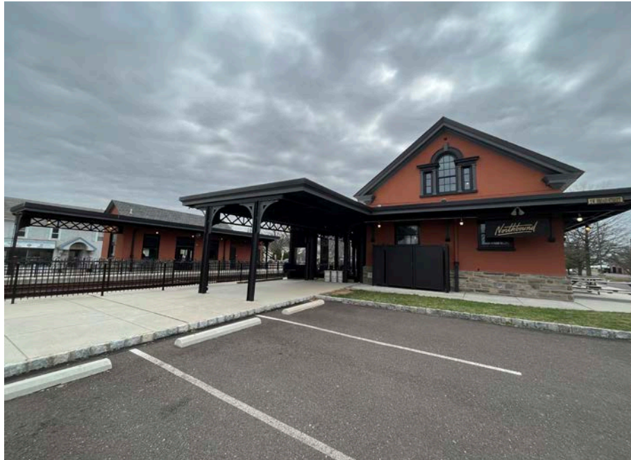
The historic train station buildings, in the heart of Souderton, have been repurposed for commercial use.
