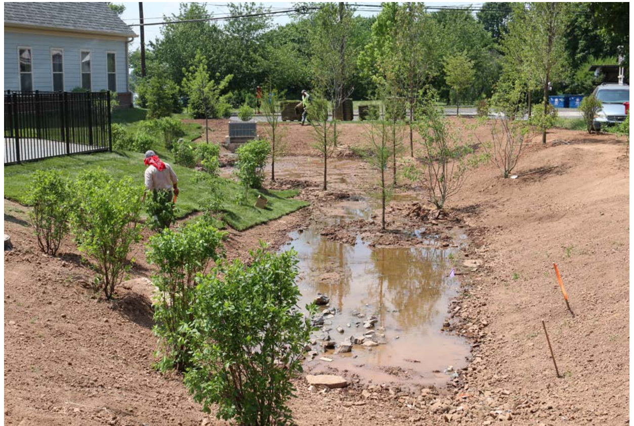
Landscaping and Stormwater Management being installed at Reliance Crossing (2016)
